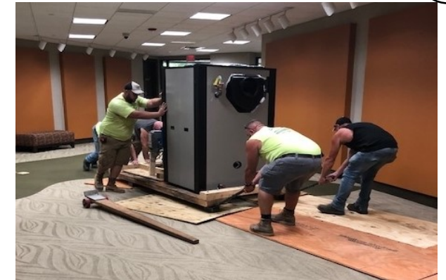
Workers bringing a new boiler into the building.
