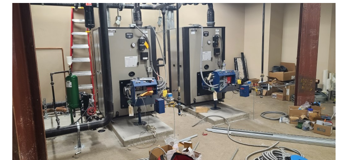
New equipment under construction
